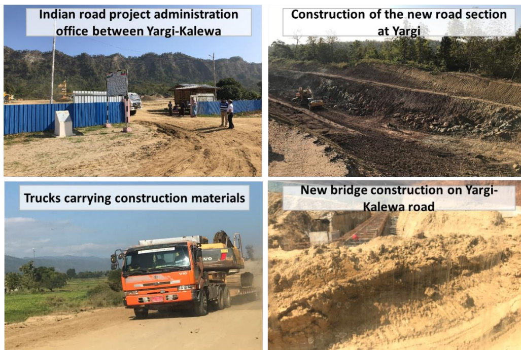
Photo 3.5. Upgrading Work on the Kalewa–Yargyi Section
